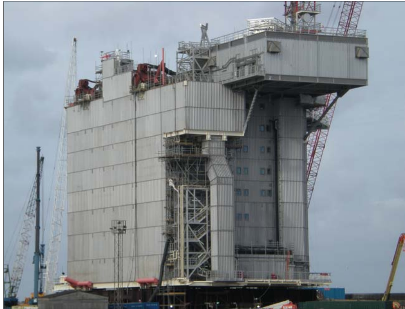
Fire and Blastwall Installation
