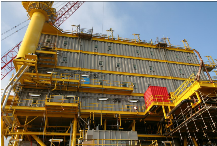
Fire and Blastwall Installation
