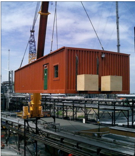
Fire & Blast Rated Calciners Module 21m x 6.6m x 3.8m high – 70 tonnes
