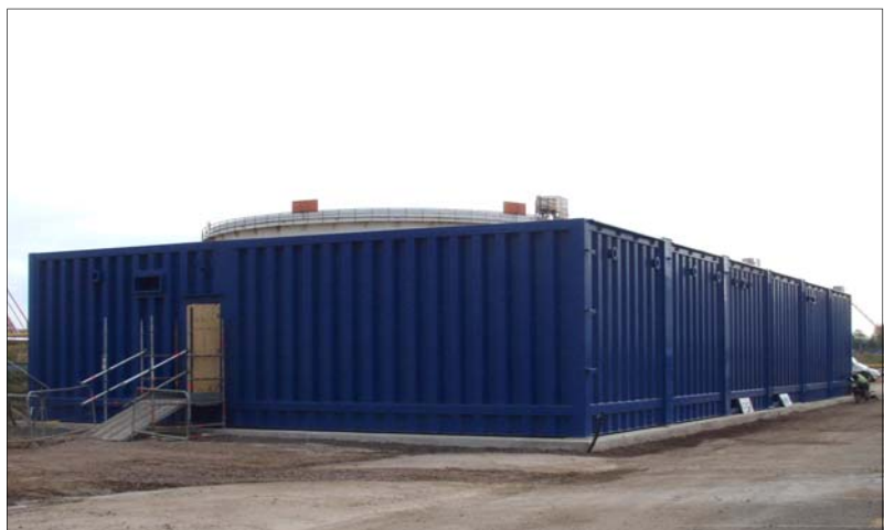
Fire & Blast Rated Module at UK Refinery
